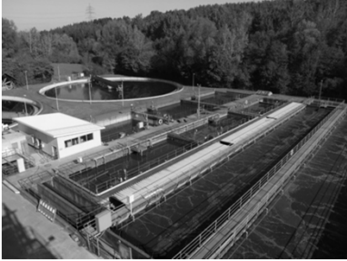
Aeration of BNR/ENR Processes
