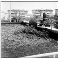
Mechanical (surface) aerators of activated sludge process treating wastewater
