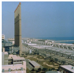
Reverse osmosis (or desalination) water treatment plants, like this one, are often located close to the ocean
